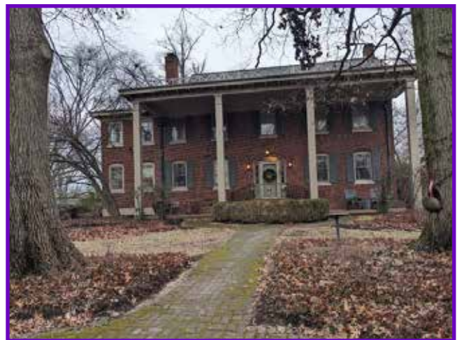
The Goosman House at 460 Hilltop Lane built in 1928 or 1929 by Dr. Goosmann.
